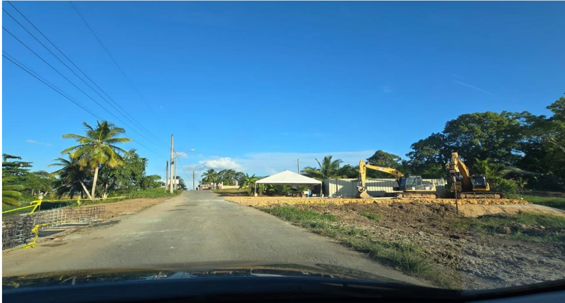
Road and bridge works underway on St John's Branch Trace.
